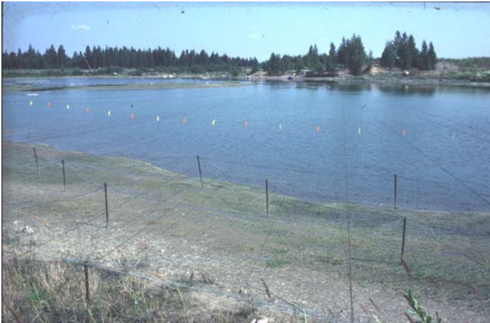
Covering and filling the ponds
